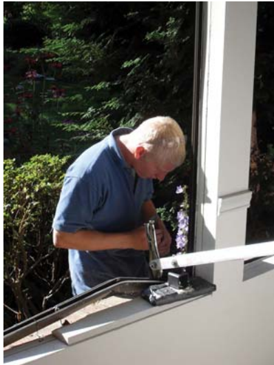
All of Penguin's installations are completed according to InstallationMasters guidelines and employees are encouraged to make time for the details.
