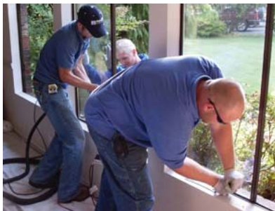
A clear advancement path helps Penguin's installers know the exact steps they must take to be promoted into a lead installer position. Crew leaders can also work their way up to field inspector, the position responsible for putting the final stamp of approval on each and every installation job.
